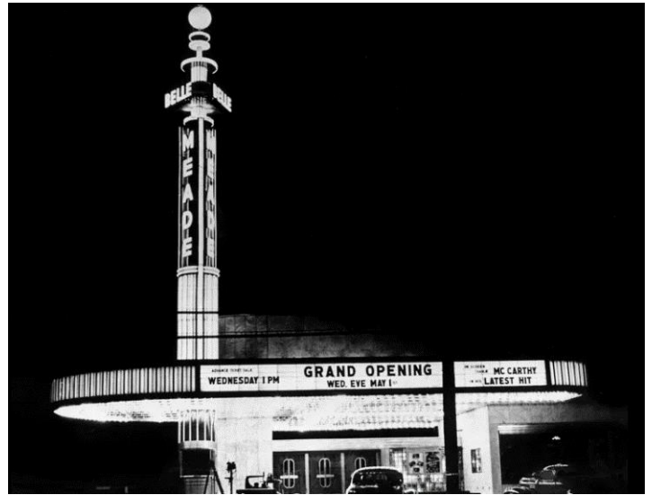
The new Belle Meade Theater is all illuminated on a spring night in late April of 1940 as the final touches are being made for the grand opening on May 1. | Credit: The Tennessean
